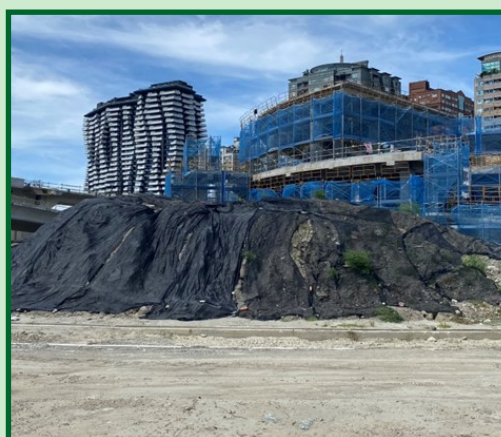
Dust net laying
