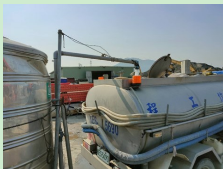
Extract water from the sedimentation tank for construction site watering and recycling (Tamjiang Bridge)
