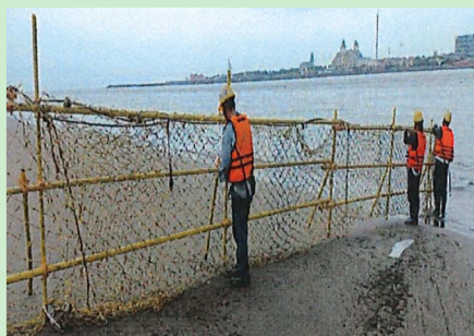
Wetland alternative fencing reduces interference to wetland
