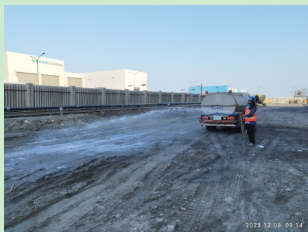
Sprinkling recycled water to suppress dust (Taichung Power Plant)
