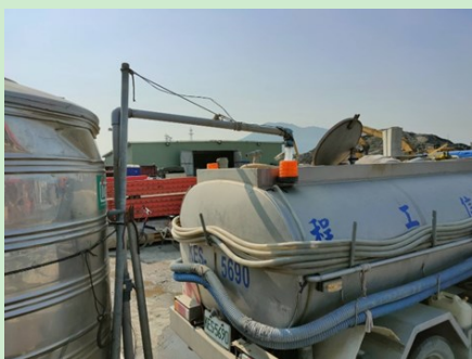
Extract water from the sedimentation tank for construction site watering and recycling (Tamjiang Bridge)
