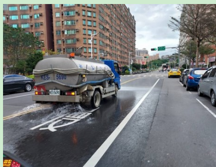
Extract water from the sedimentation tank for construction site watering and recycling (Tamjiang Bridge)
