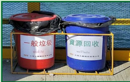
Garbage storage equipment and garbage sorting at the construction site
