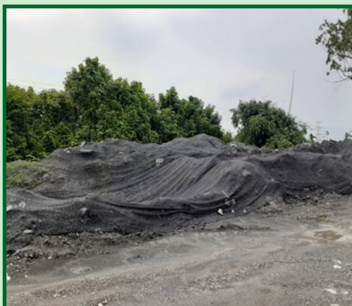
Dust net laying
