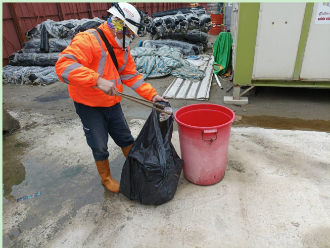
Picking up rubbish in the work area
