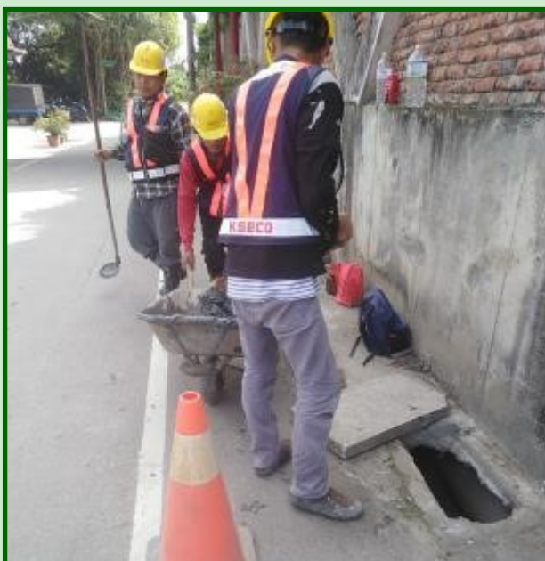
Work area drainage ditch cleaning
