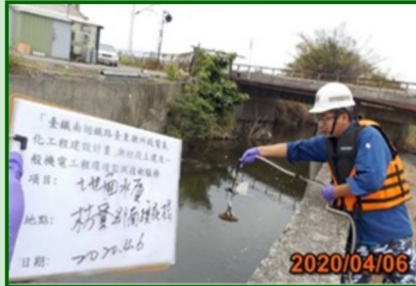
Surface water quality monitoring
