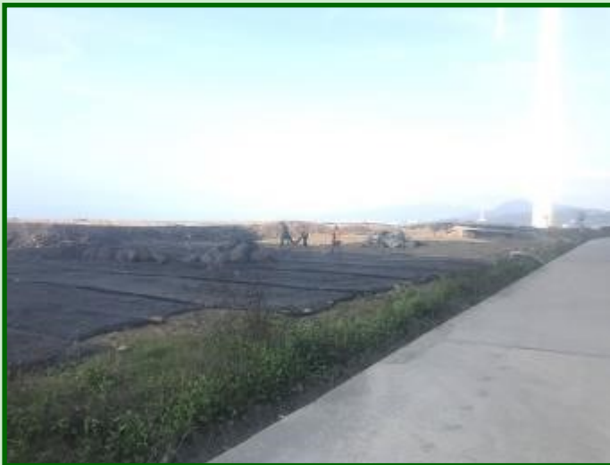
Dust net laying
