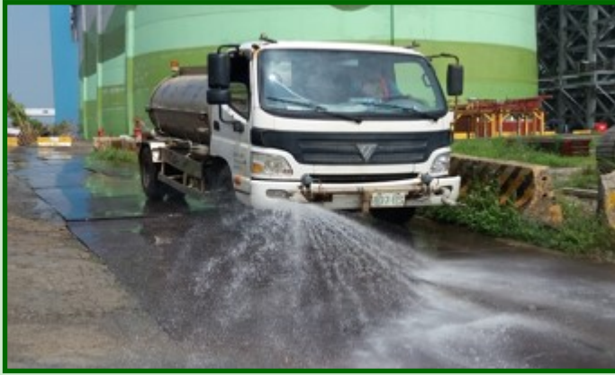
Washing and sprinkling water on the road in the work area
