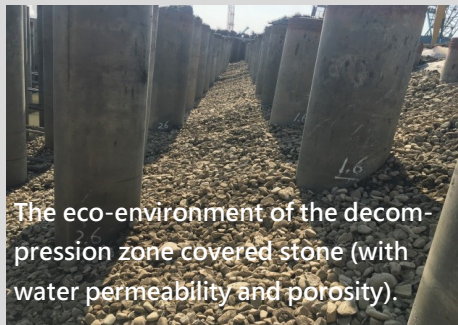
Decompression zone (with water permeability) + foundation pile + stone (with porosity)
