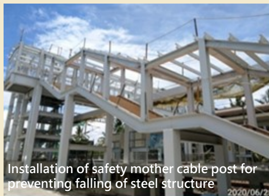
Safety protection for workplaces with a height difference of two meters
