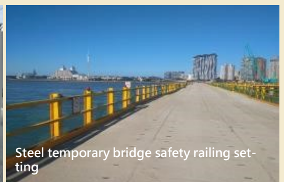
Safety protection for workplaces with a height difference of two meters
