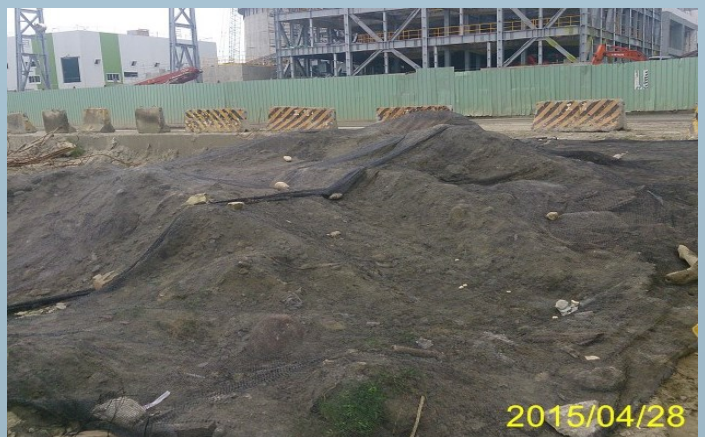
堆置土方鋪設防塵網防止揚塵
